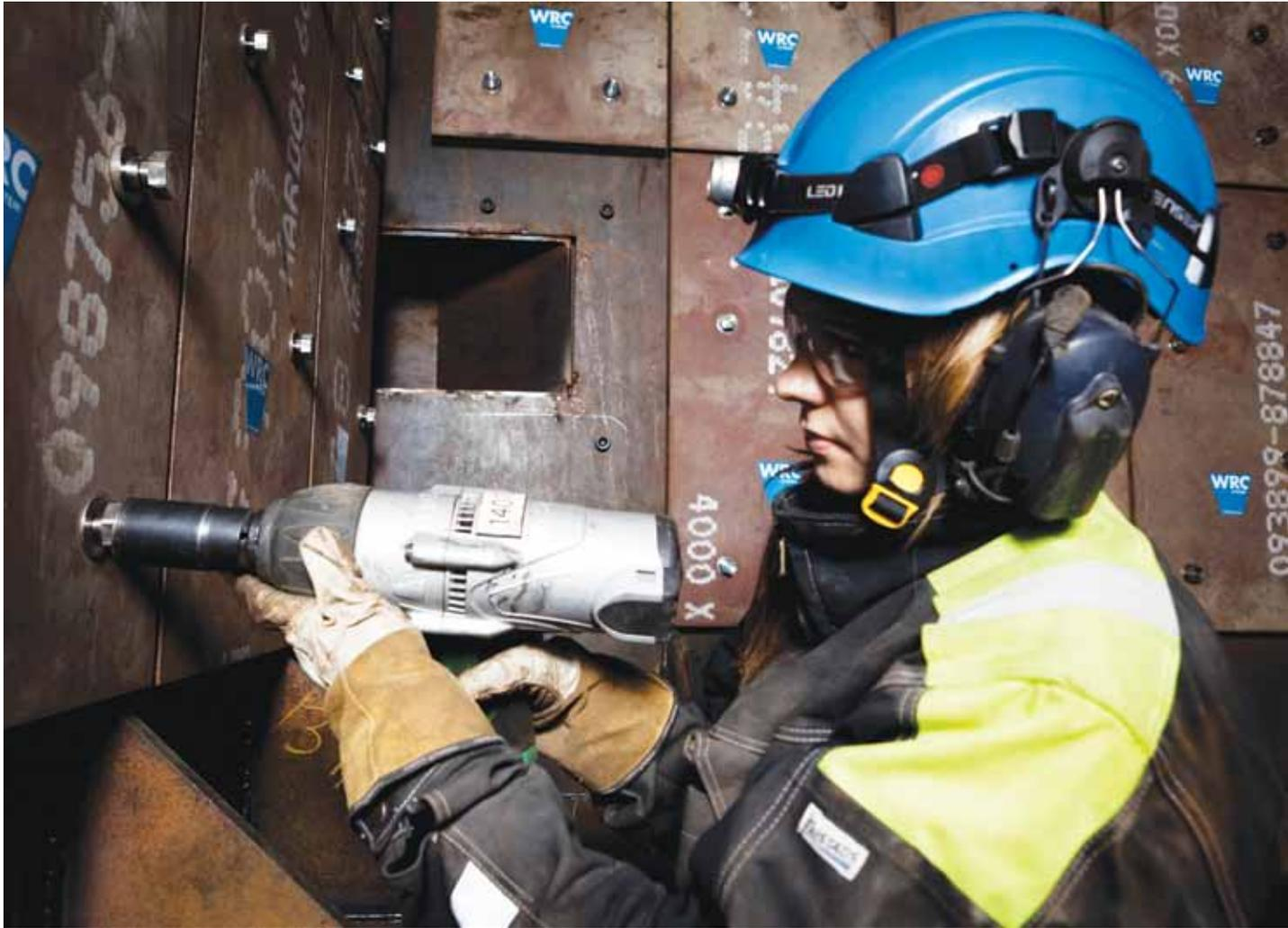
Installation of WRC socket screw.
